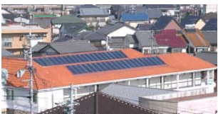
Care home (Komagane) Collector92m 2 Storage tank1.1m 3 Space heating and Hot water for spa and shower. Day-care and Short period staying facility for old people.
