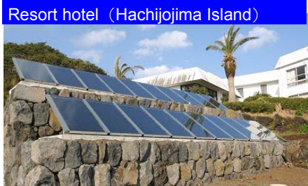
Resort hotel (Hachijojima Island) Collector40m 2 Storage tank5m 3 For the shower and hot water supply. Extremely salty environment required anti-salt treatment.
