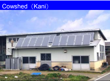
Cowshed (Kani) Collector40m 2 Storage tank1.5m 3 Hot water to wash Sanitary Plumbing for Milk..
