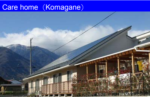
Care home (Komagane) Collector92m 2 Storage tank1.1m 3 Space heating and Hot water for spa and shower. Day-care and Short period staying facility for old people.
