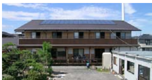
Care home (Komagane) Collector92m 2 Storage tank1.1m 3 Space heating and Hot water for spa and shower. Day-care and Short period staying facility for old people.
